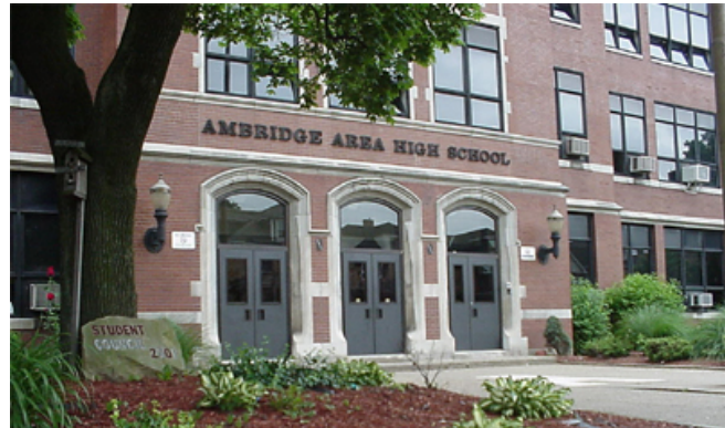
Existing Ambridge Area High School
